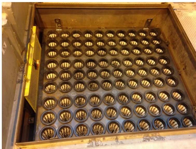
Figure 4. First converted Vibrair chamber.
