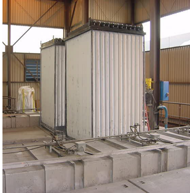
Figure 2. Filter block with 12 pocket bags.
